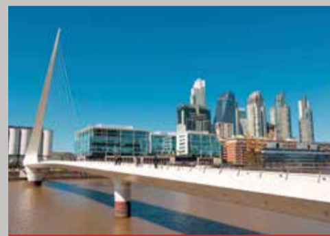
Puerta de la Mujer, Buenos Aires, Argentina: The bridge has two fixed sections and a movable one in the middle that rotates around a pylon to resemble a couple dancing the tango.
