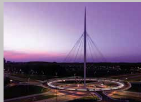
Hovenring, Eindhoven, Netherlands: This is a suspended roundabout, 72m in diameter, 70m above the ground, for pedestrians and cyclists.
