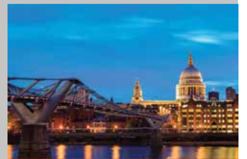
London Millennium Footbridge, London, UK: Known as the Millennium Bridge, this is a steel suspension bridge to carry pedestrians over the River Thames.
