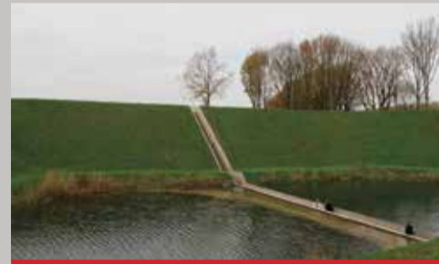
Moses Bridge, Halsteren, Netherlands: This "invisible" bridge is built beneath the waterline so that pedestrians appear to be walking on water.
