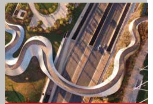
BP Pedestrian Bridge, Chicago, US: This serpentine bridge connects Millennium Park and Daley Bicentennial Plaza. It also acts as an acoustic barrier against the traffic noise from Columbus Drive.
