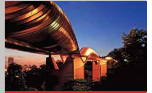
Henderson Wave Bridge, Southern Cordillera, Singapore: This bridge's distinctive wavy structure, which stands 36m above the road, is made of steel and wood.
