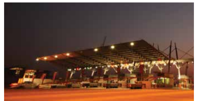
The Diamond Hill Plaza (managed by TRAC) started using solar power as an alternative energy source in September 2014.
