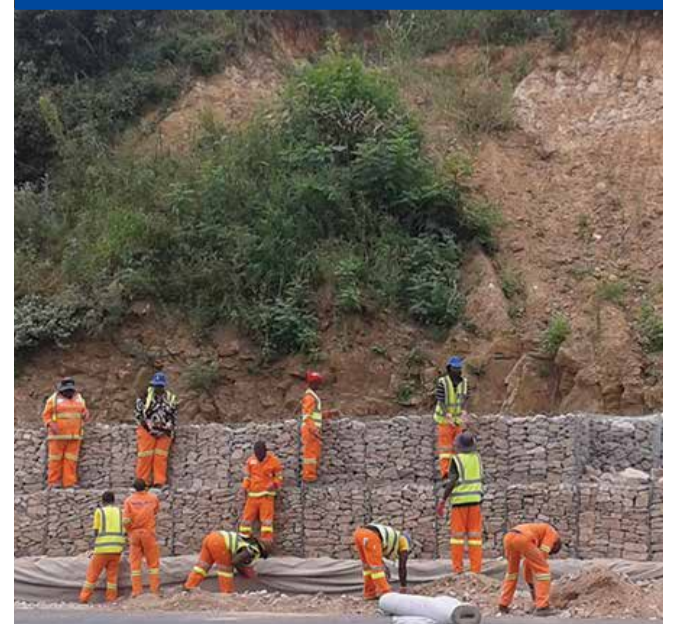
On the N2 between Murchison and Marburg, the use of RA was specified at 40%, resulting in 40% less aggregate to be crushed.
