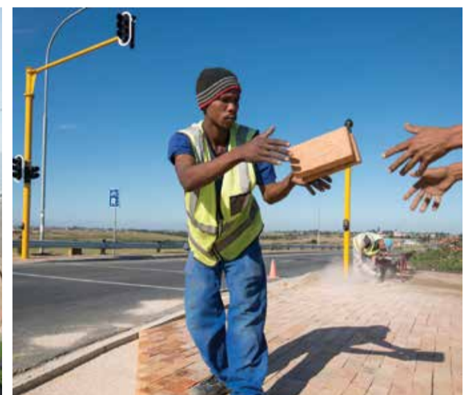
Local labour was used in the laying of kerbs.
